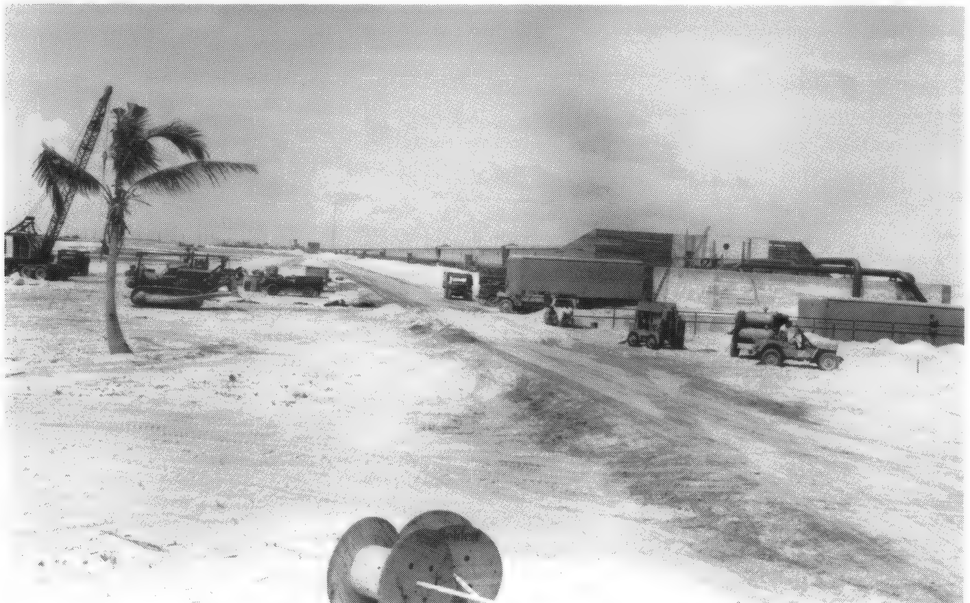
FIGURE 5-28. KRAUSE-OGLE HELIUM BOX FROM MIKE CAB TO STATION 200
